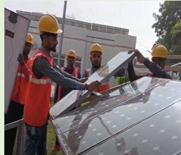
Training on Solar Plant Installation
