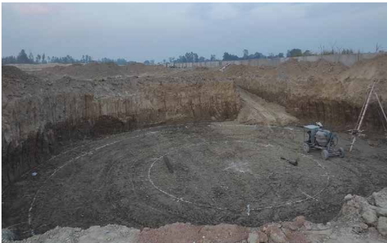
Figure 20: Construction site of the CBG plant in Misrikh
